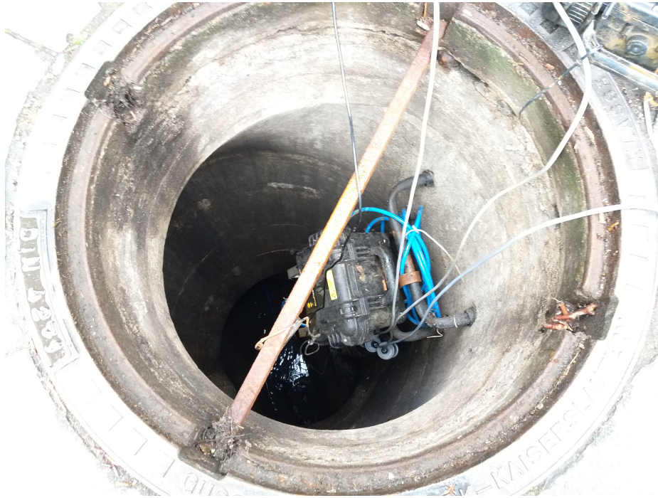
Figure 2.5: Gws box inside the sewer pipe. This is one way the data was collected.
