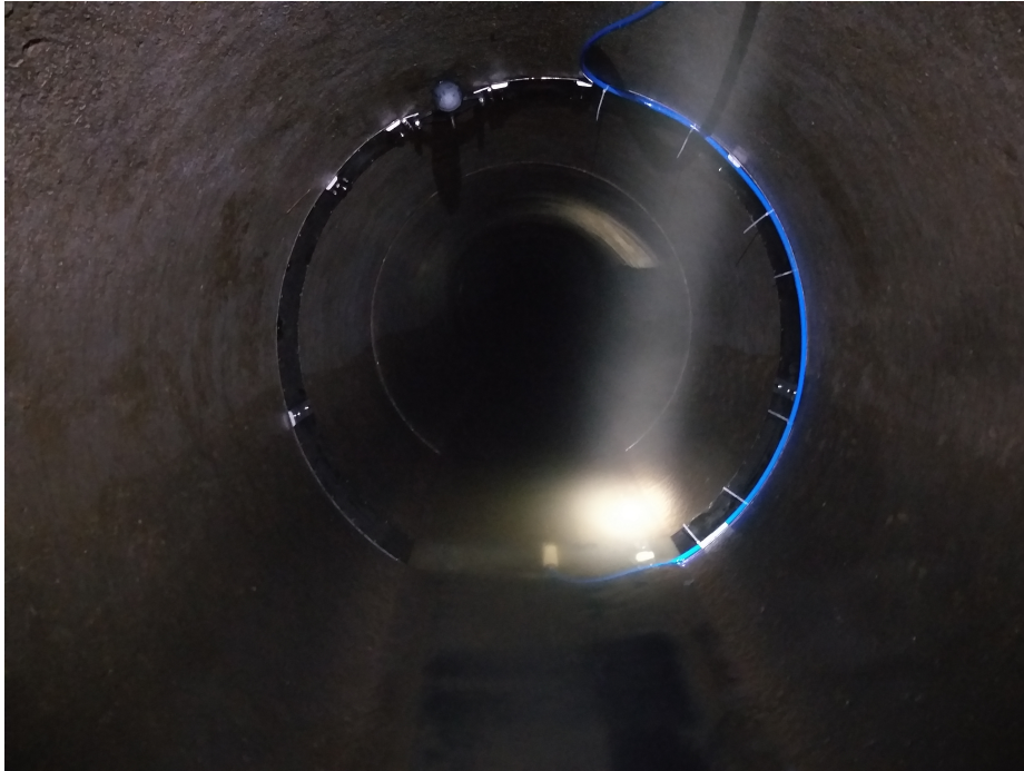
Figure 2.2: Sensor inside the sewer pipe connected to the NivuFlow Mobile Box.
