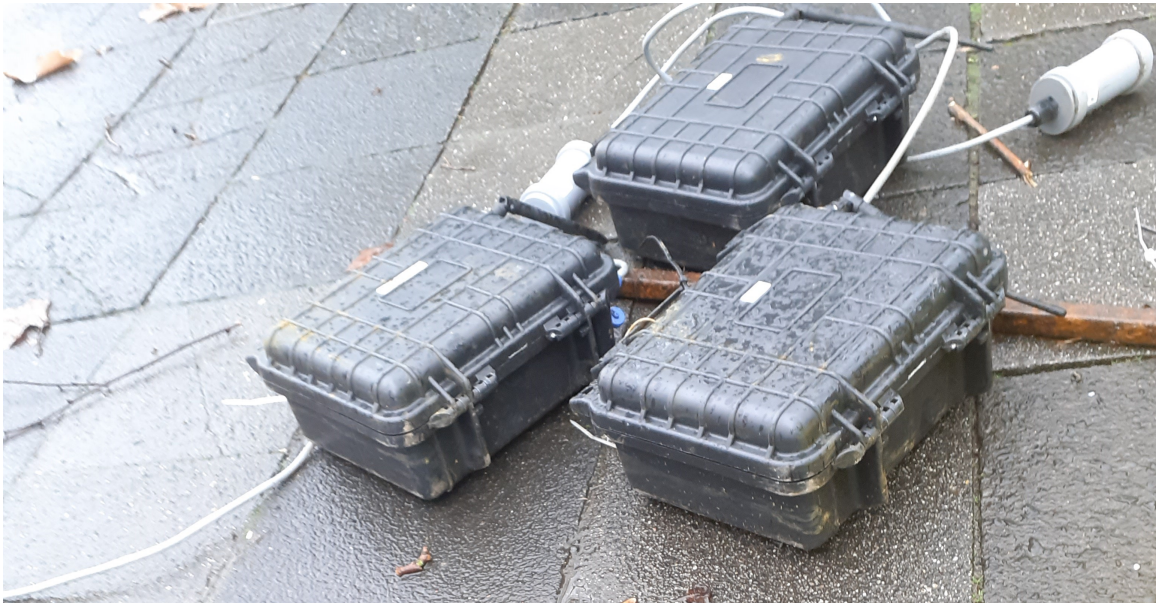
Figure 2.3: Boxes containing all the electrical elements.
